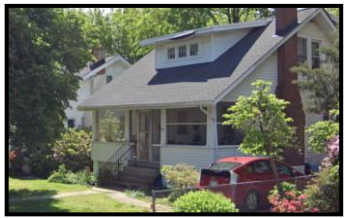
Typical Aurora Highlands House on 23 rd Street, ~25' tall
