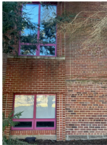
4) Entry canopy missing, limestone trim missing at center portico, and front steps / doors replaced – new work is inset within the original masonry opening
