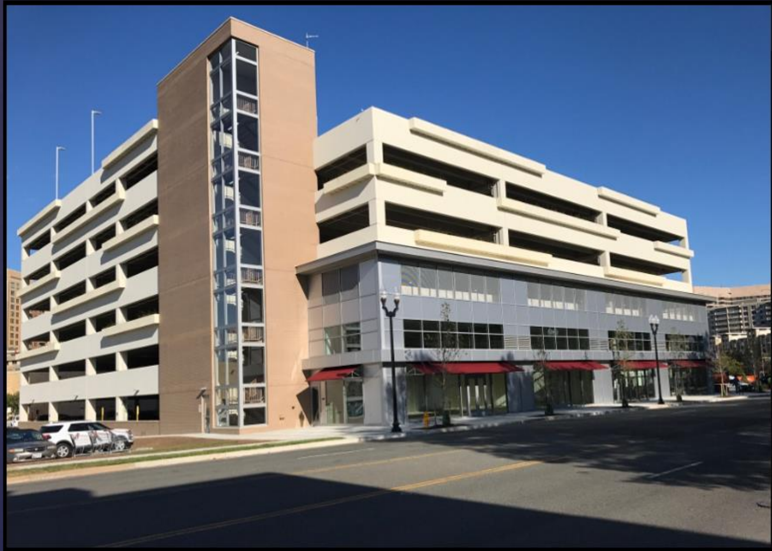
Building D- 15 th Street View at Grant Street
